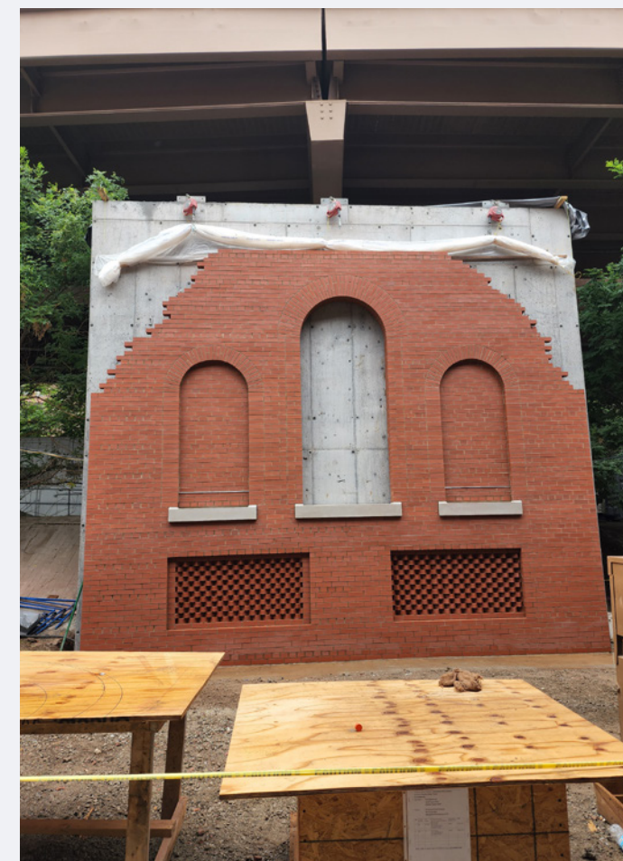
Replication of the historic infill wall. Photo Credit: Jacqueline Bascetta.
