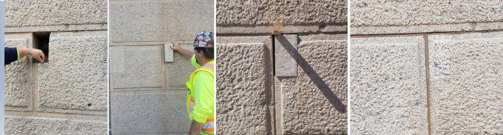
Matching Dutchman materials to the existing. Photo Credit: Jacqueline Bascetta.
